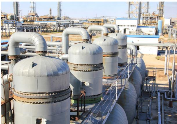
**Figure 3.** A typical multi-stage FIBER FILM Contactor and separator system treating light crude oil in a stick built unit.
